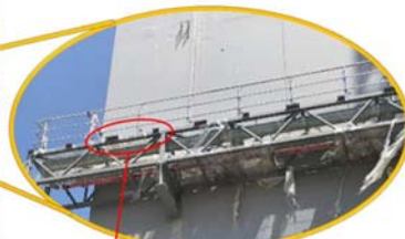
Mounting points for façade
